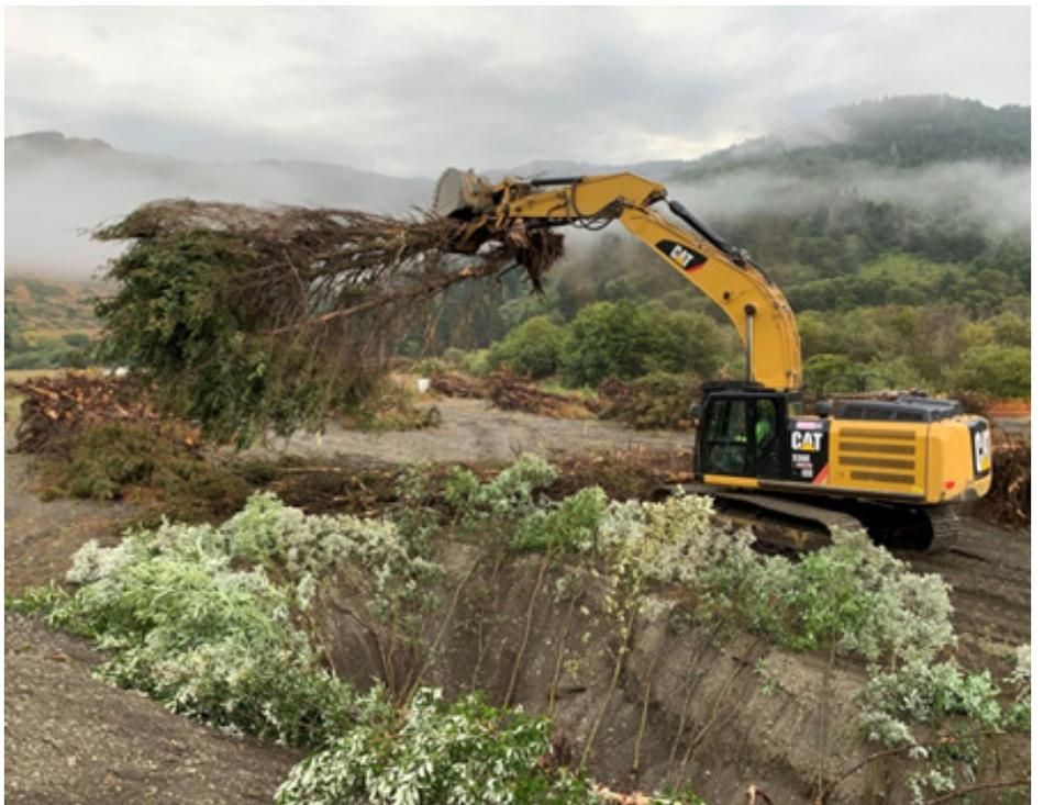
*Placing douglas-fir removed from Prosper Ridge grasslands restoration site in a lower river willow structure.*
